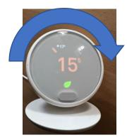
To decrease the set temperature then turn the outside ring of the thermostat anticlockwise. The large number in the middle will decrease.
